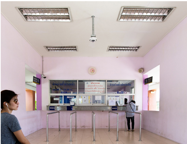
Example 5: Installation of Oncam Evolution 12 Outdoor in ticket hall of Hua Lamphong station in Thailand
